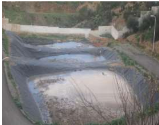
Leachate lagoon basins at the landfill Technical Center of Souk-Ahras city.
